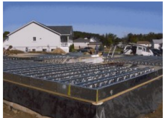
Photo # 3 – Floor Framing
